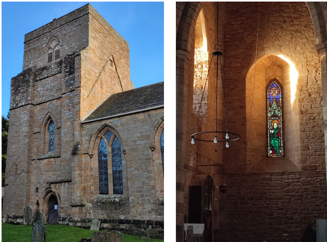
Figure 1. St Mary the Virgin, Blanchland, on 11 February 2023 (left) and 21 January 2023 (right).
